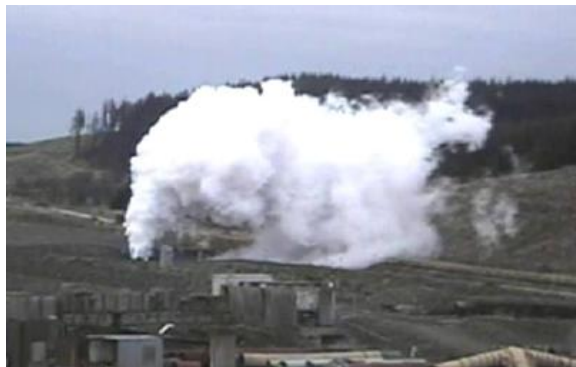
Bent-over plume, no CO 2 re-entrainment
