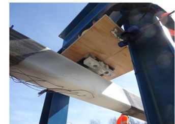
SHS underside after 200s release
